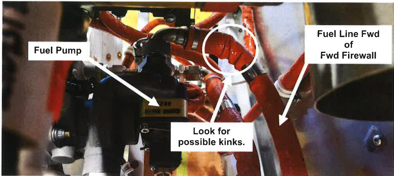
Figure 8.2.3 – Fwd Fuel Line Inspection
